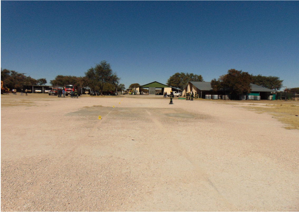
Figure 5: View of the A2 – MBE tracks as it was approaching the engine run-up area prior to encroaching onto runway end safety area.
