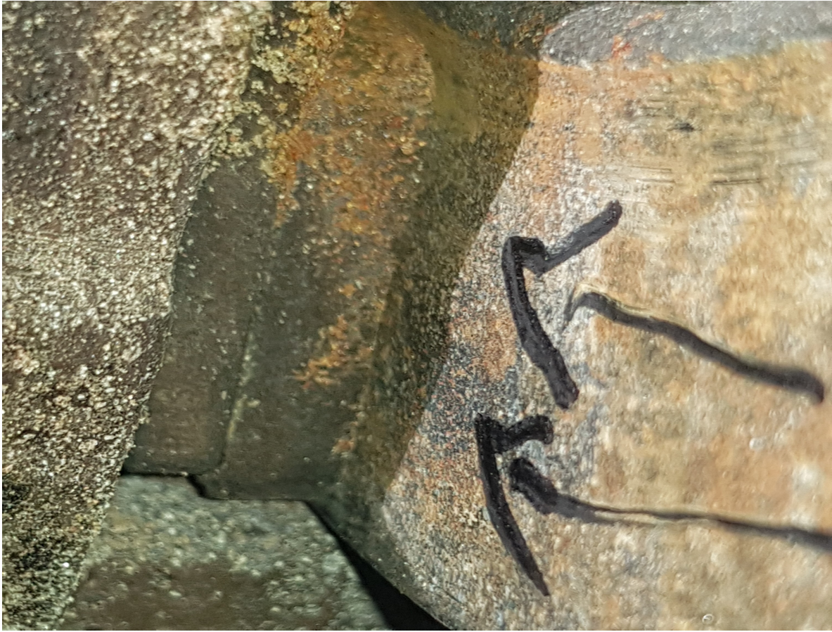
Figure 7a: Close view showing left main gear brakes pads engaged on the disc.
