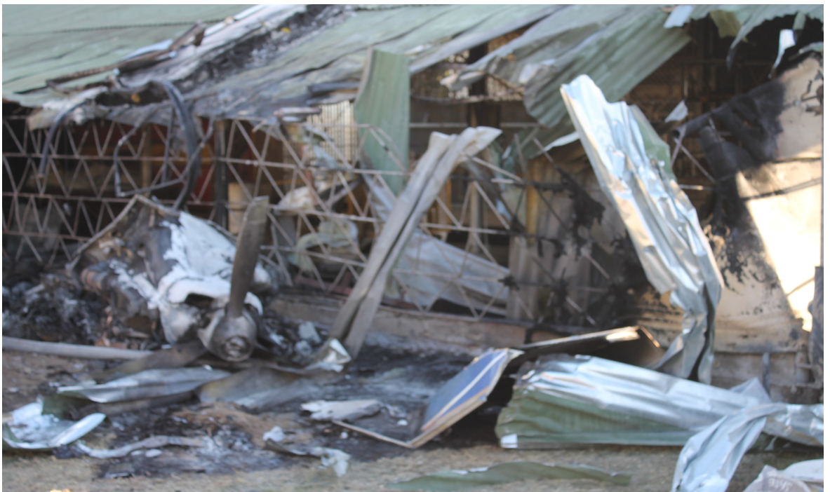
Figure 2f: View of aircraft nose with propeller blades next to damaged side wall of the farm shed.
